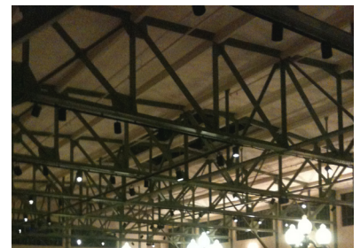
Example of open steel beams
